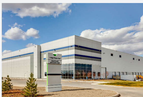
High Plains Building 10 in Calgary, Canada, which received the CoStar 2024 Impact Development Award
