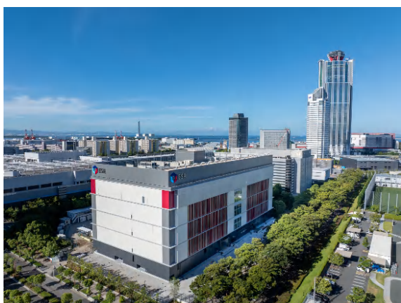
The ESR OS1 Data Centre in Osaka, Japan, which we invest in through the ESR Data Centre Fund
